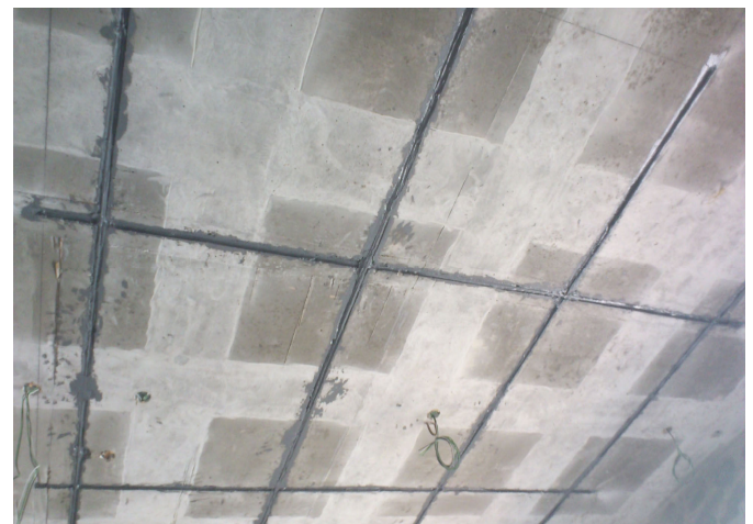
Build Rod HS 16, install under Slab
