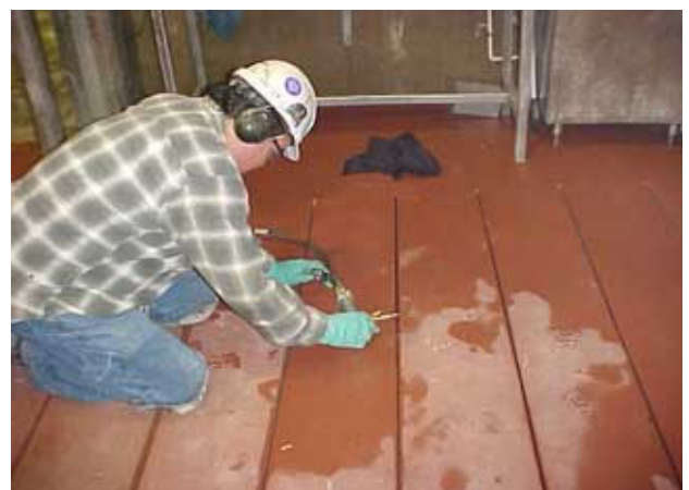
Build Rod HS 16, install on top Slab
